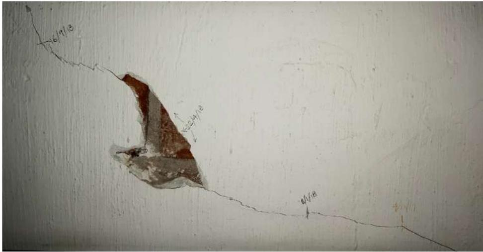
Figure 17: Section of a dated fissure passing behind a shelf in Elena's living room.
